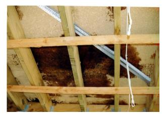
The photograph on the left shows the effects on an area subjected to wetting, which was floored with ordinary particleboard and insufficiently protected with a poorly applied membrane.
